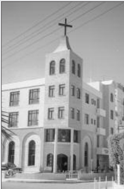
The new facilities of the John Calvin Centre.
