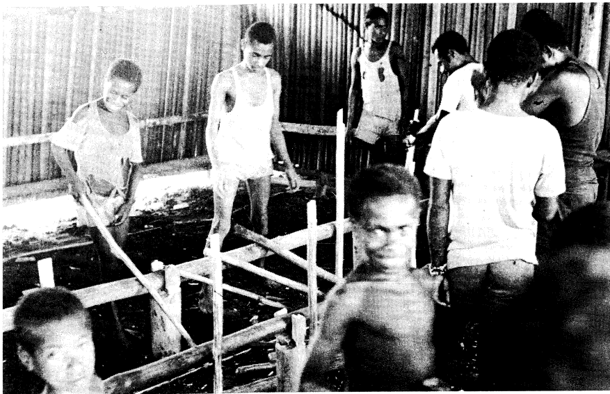
"Starting at the bottom with frame work for benches and desks."
