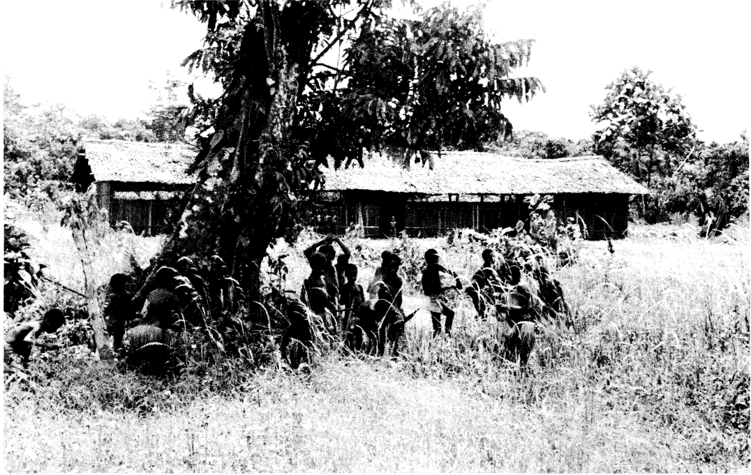
"Clearing ground in front of the new school in Mangelum."
