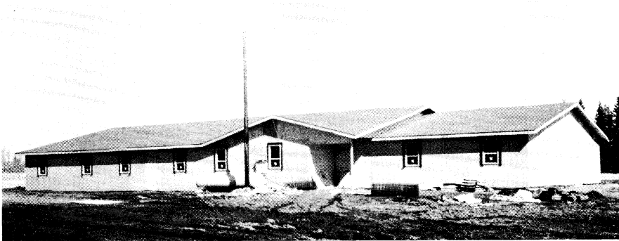
Edmonton's school building under construction.
