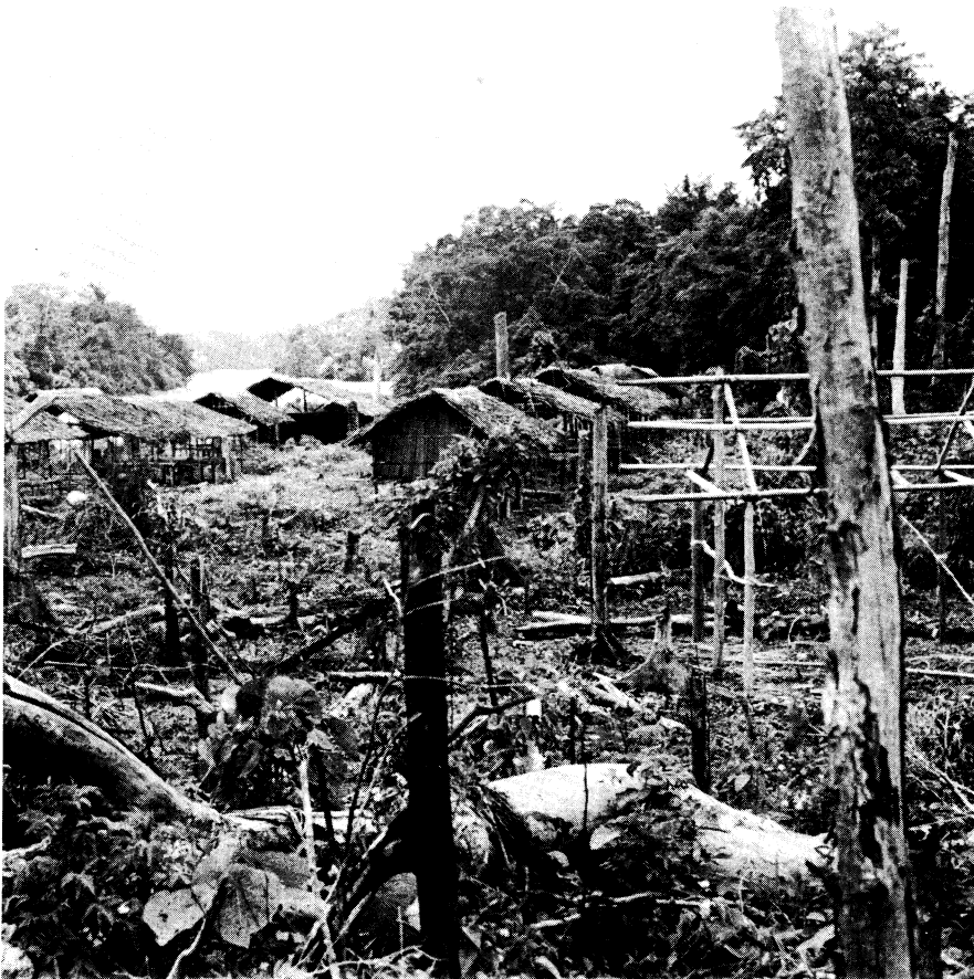
The new Heyokubun under construction.
