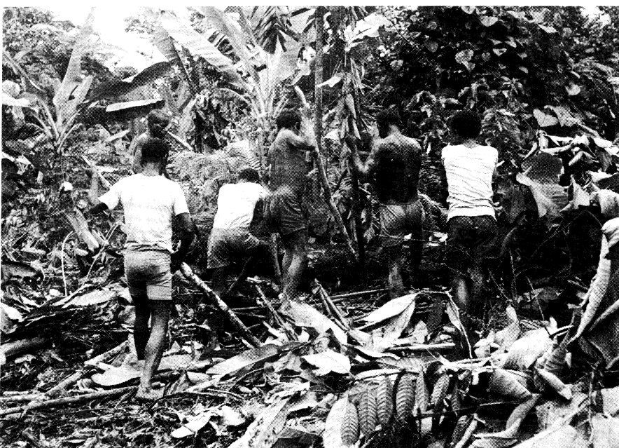
Clearing the jungle for the new strip in Manggelum.
