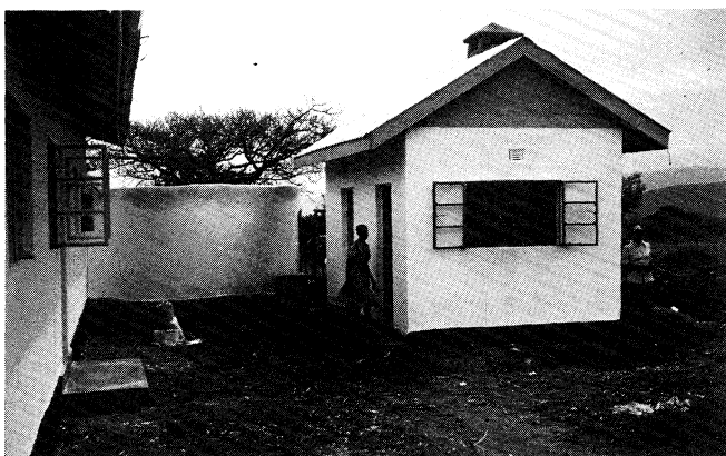
View of cookhouse and large water tank at back of home. The tank supplies all of the home's water.
