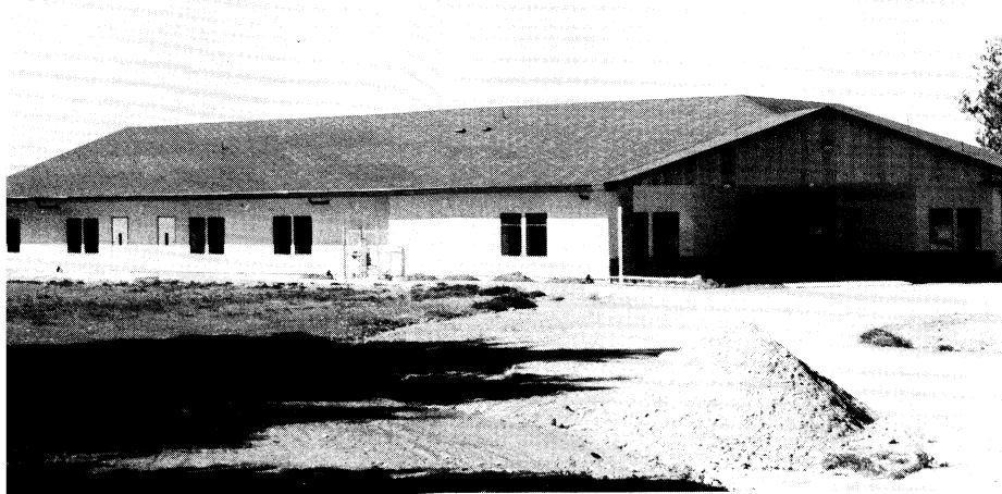
Credo Christian Elementary School, Langley, BC. The first phase of the school building.
