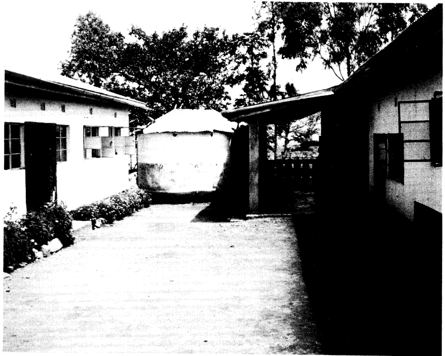
l-r: Girls' dormitory, kitchen verandah, and the dining hall
