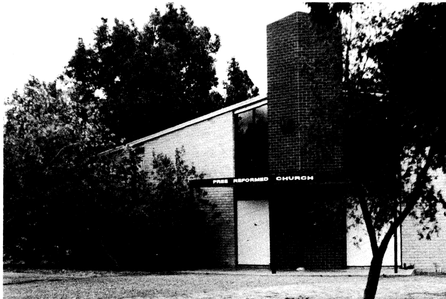
Armadale's church building where Synod is held
