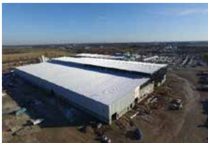
Plant #3 – Under Construction
