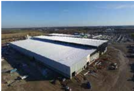
Plant #3 – Under Construction
