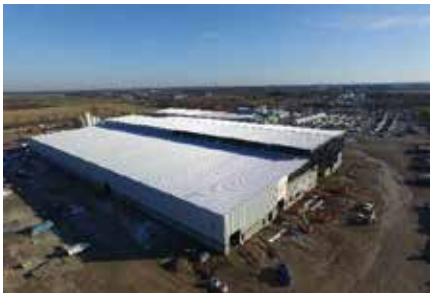
Plant #3 – Under Construction
