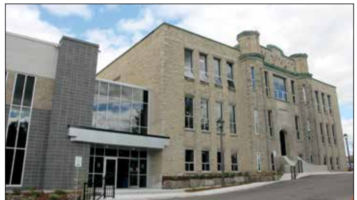
Old and new blended together: the renovated, historic high school build in 1927 in Fergus (right) with a new entrance and full size high school gymnasium (left) is the new home for ECHS
